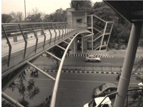
Pedestrian Bridge, New Delhi
