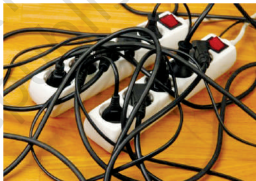
Fig. 1.29: Overloaded extension cords
