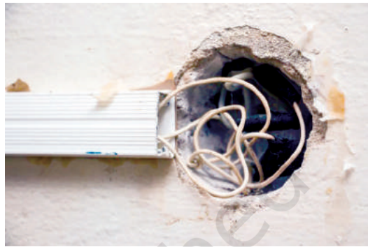
Fig. 1.28: Be careful of exposed cables
