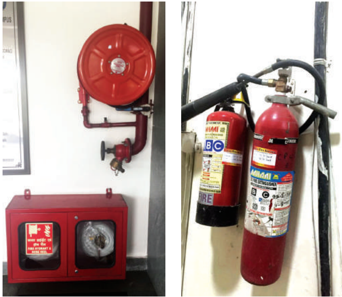
Fig. 5.1(a,b) Fire extinguishers
