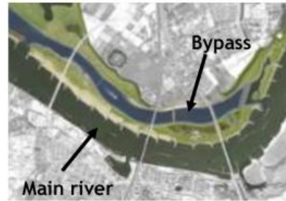
Figure 1: Aerial overview of the bypass and main river.
