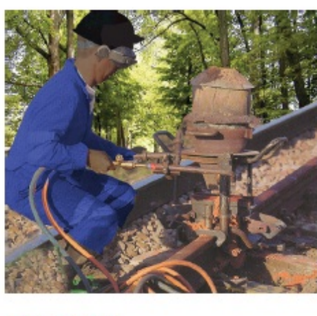
Figure 3.11 Thermite process for joining railway tracks
