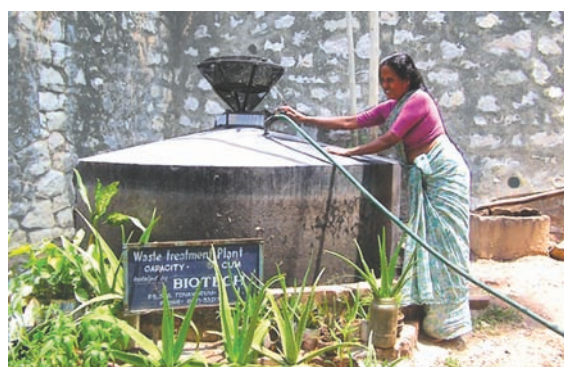
Fig-8 : Bio gas plant
