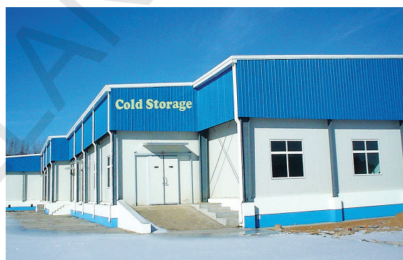
Fig-28 Cold storage unit
